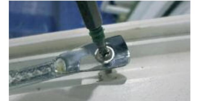
**5** Then position the sash between the parting bead and the external frame liner but leave the right hand side so that you can see the screw. Pull down the sash cord and hook it onto the screw and tighten. Using a 1mm gauge of plastic laminate, or similar material, as in item 6 (installing spring balance sashes) and slide the sash into place.
