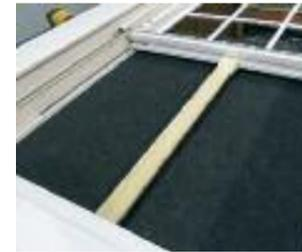
**7** Using the brace cut earlier push sash to upper position and place under sash.
