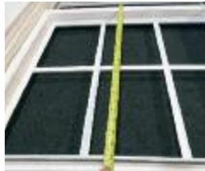
**4** Measure the height of the sash from the top to bottom rail, work out the distance from bottom rail to cill, then cut a wooden brace and pad the brace at either end so as not to damage the sash or frame.
