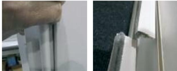
**1** Remove right hand side of staff bead, this should be left partly unclipped, then remove right hand side of parting bead.
