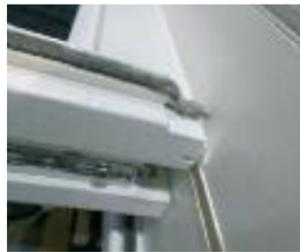
**6** When fitting the sash you will notice that the flipper weather seal is inverted and catches on the plastic channel on the frame. To help ease the sash into position you will need a 1mm thick gauge of plastic laminate, or similar material, to slide between sash and frame.
