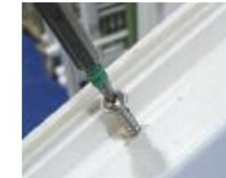
**3** Loosen off screws on the side of the sash but do not remove.
