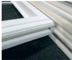
**5** Offer the top sash up to the frame, slotting the left hand spring groove on the sash over the left hand spring. Then place the right hand spring in the spring groove on the sash. Then replace the sash into the frame.
